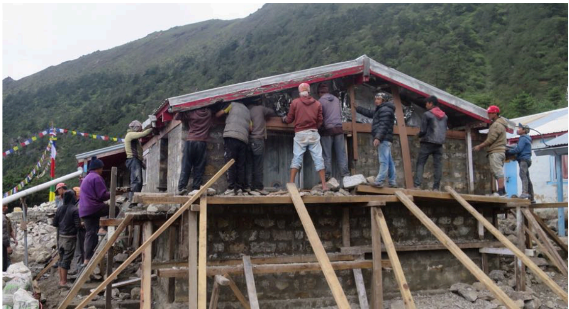
Figure 4: Builders setting up lentil tie around the main building
