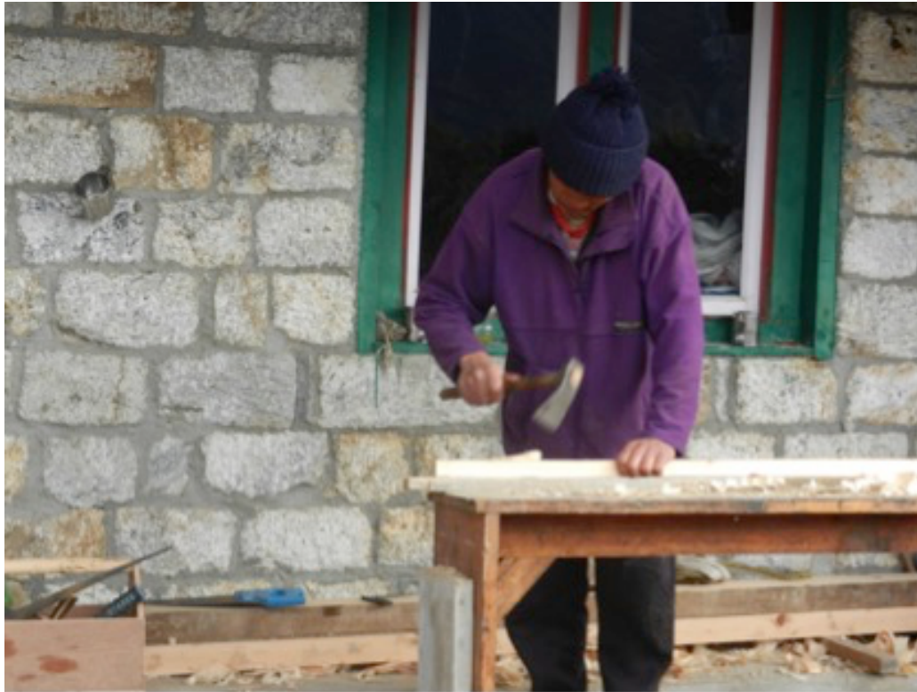
Figure 6: Carpenter making chairs from reusing wood used for supporting the building during construction
